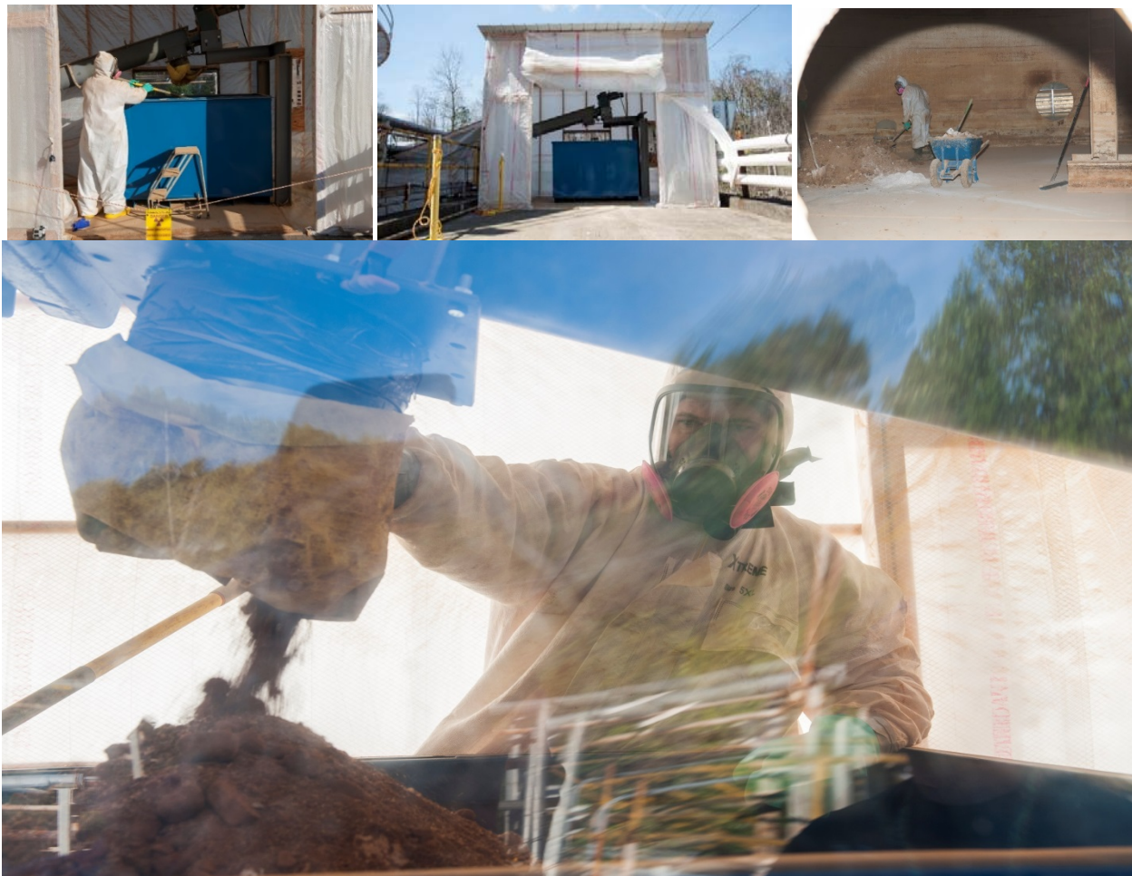
Figure 7. Sludge Removal Inside Tank and Box Filling Operations.
