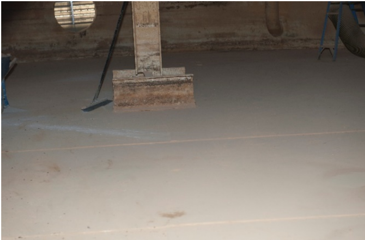
Figure 9. Tank Inside Surface After Sludge Removal and Ready for Structural Integrity Inspection.
