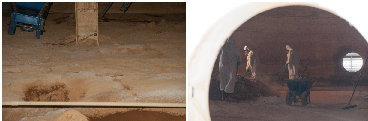
Figure 8. Before and After Sludge Removal Inside Tank.
