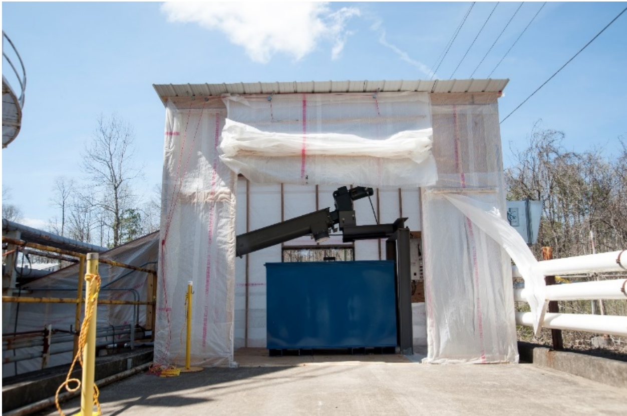
Figure 4. Box Containment Structure Showing Auger Discharge Shoot.
