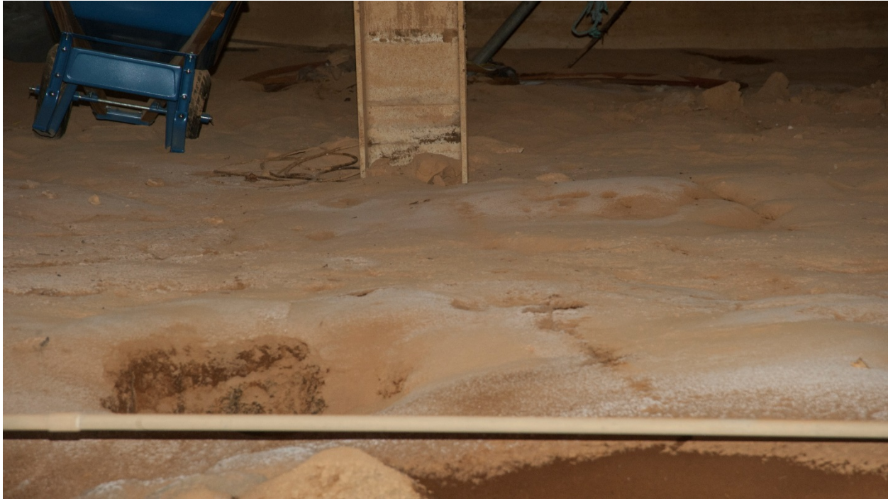
Figure 2. Inside View of Tank Prior to Removal of Sludge.
