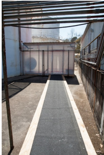
Figure 5. Elevated Walkway to Boundary Control Station to Allow Work When Dike Contained Water.
