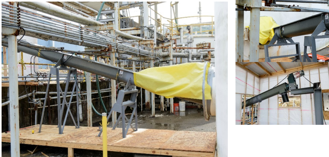
Figure 6. Construction of Sludge Auger Conveyor System.
